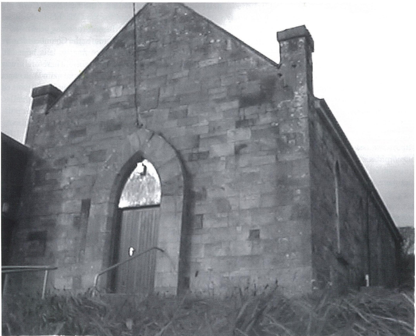
The former Presbyterian church on the Castlebar road, now used as a youth centre
